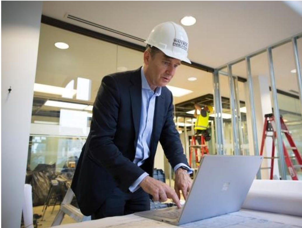
Adam Waterous, CEO of the Waterous Energy Fund, during construction of his firm’s Calgary office in 2017. Photo by Todd Korol for National Post files
