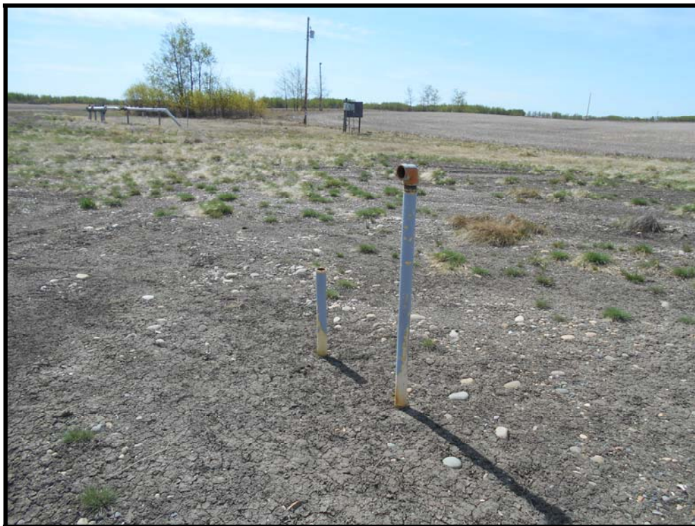
Pipe stems northwest of well centre – potential underground tank
