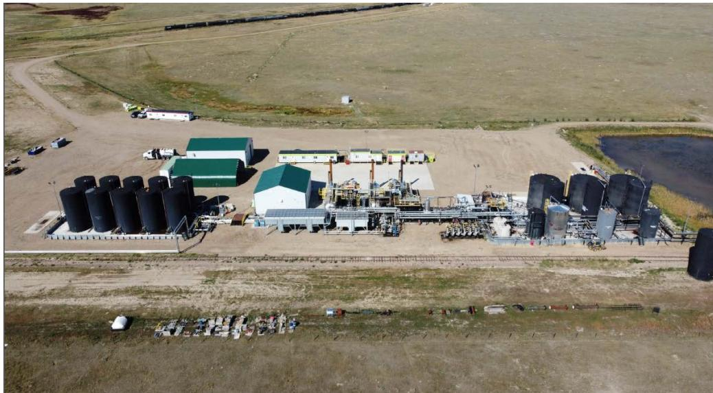
Echo Refinery's operations include the UMO processing plant, UMO inlet tank farm, processing/sales tank farm and a surface water retention pond located adjacent to the eastern berm.
