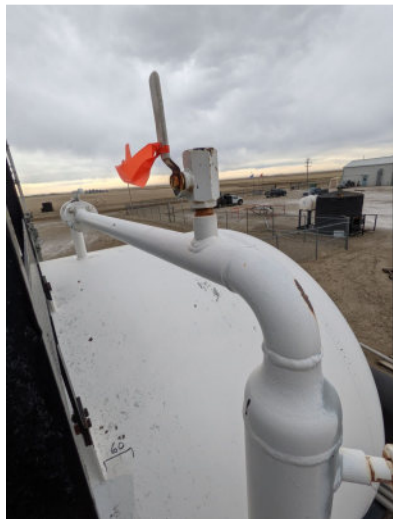
Unplugged valve on liquid level piping
