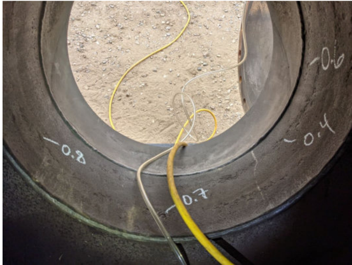
Manway nozzle corrosion
