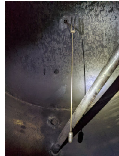
Float is contacting overflow piping
