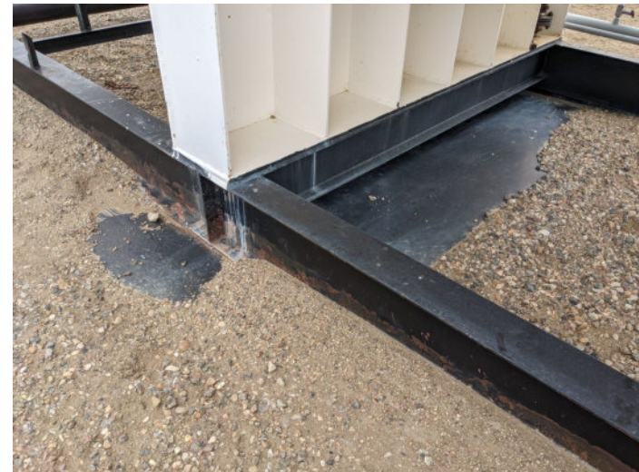
Saddle is welded to skid
