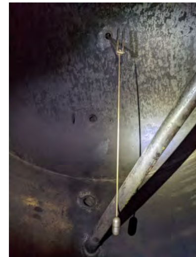
Float is contacting overflow piping
