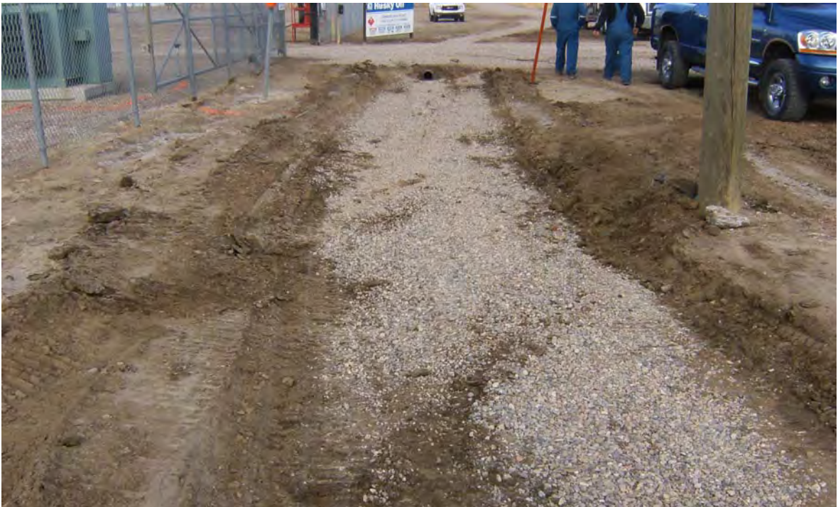
Photo 2: View of gravel swale and culvert under access to plant, looking north.
