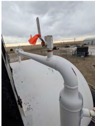
Unplugged valve on liquid level piping
