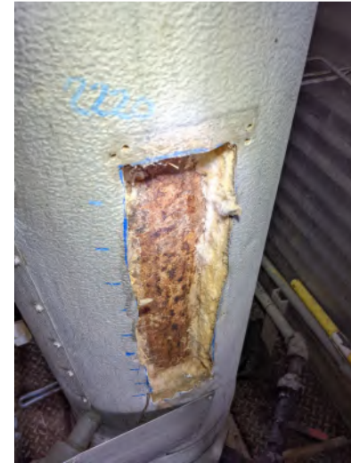
Non-measurable corrosion at CML Port
