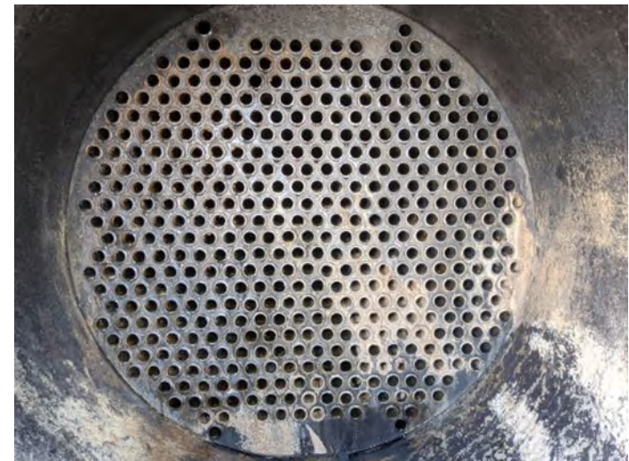
North End - minimal solid build up in tubes.
