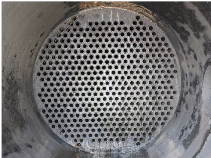
South end. minimal solid build up in tubes.
