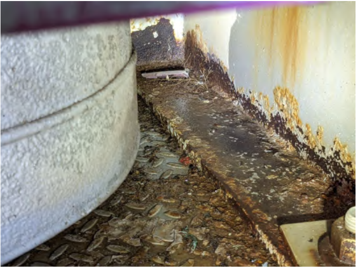
Missing Anchor Bolt
